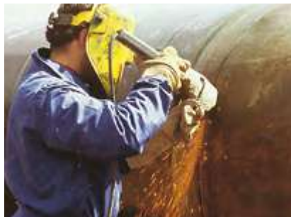
Creation of traces on reinforced concrete.
